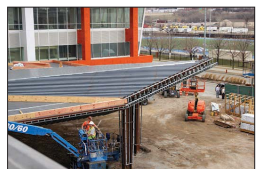
Unfinished main entrance in to hotel
