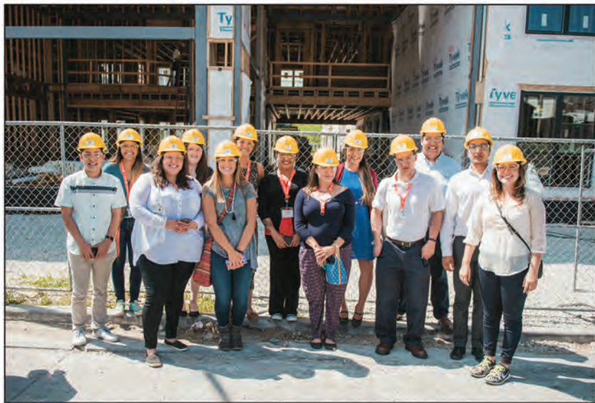
Greenfire Management Services gave students a tour of one of their current projects, River House Apartments, located along the Milwaukee River. This $35 million development will contain 450 upscale residential units within four, 4-story buildings that will sit over two levels of underground parking. Each building will feature a large resort courtyard that opens to a river walk with access to the water.
