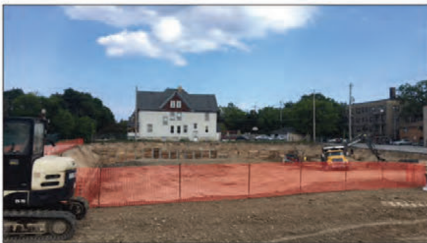
Pictured above: Progress of parking structure as of August 16, 2017.
